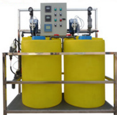
Dosing Tanks in Water Treatment Plant
